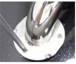
8. Attach bar to adapters using the screws included. Make sure to reattach in same position as originally set to be sure screws align properly. Tighten firmly. Slide cover ring over base and turn clockwise until properly aligned and turn to lock in place. Job complete!
